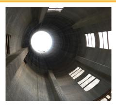
foundation and construction can begin. Concrete is placed in the forms, and the forms act as a moving die to shape the concrete. The rate of movement of the form is regulated so that the concrete leaves the form after it is strong enough to retain its shape while supporting its own weight.
