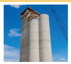
is solid concrete without voids or cavities. All surfaces are smooth and vertical, facilitating the flow of food ingredients. Slipform walls can have rigid insulation installed in the center of the concrete wall, creating a sandwich panel with concrete on all sides of the insulation, sealing it off from any exposure.
