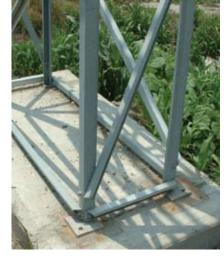
Easy bolt together galvanized steel components for ultimate strength and rigidity. High tensile strength, galvanized bolts and bardware make for a "total maintenance free unit".
