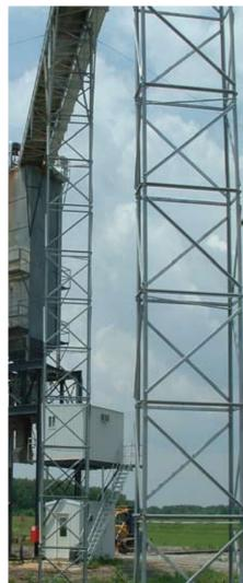
Precision Fabricated Galvanized Steel for Fast and Easy Modular Erection Without Welding, Painting or Field Alteration
