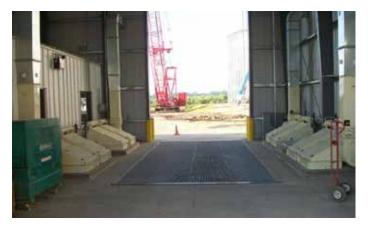
Point-of-use dust collectors capture nuisance dust while keeping product with the grain stream.
