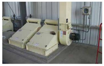
Point-of-use dust collectors allow for easy maintenance.
